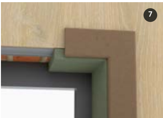
Door finish with MDF and door frame
