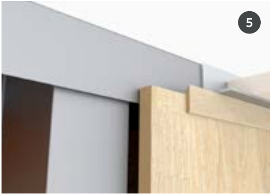
Ceiling finish with flexible interior and external corner profile
